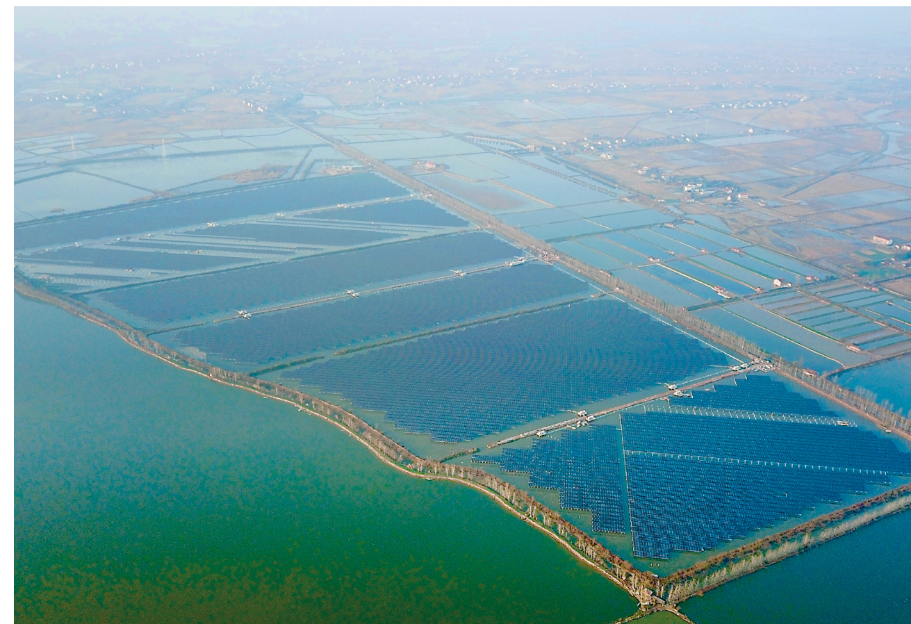
常德兴阳80MW渔光互补项目 Changde Xingyang 80MW fishing-PV complementary project
